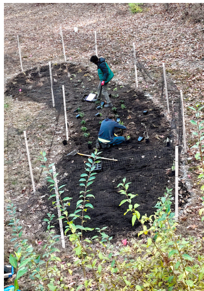
◀ Crewmembers from Howard EcoWorks install a septic garden in 2023. This project was funded by the Chesapeake Bay Trust and Howard County.
